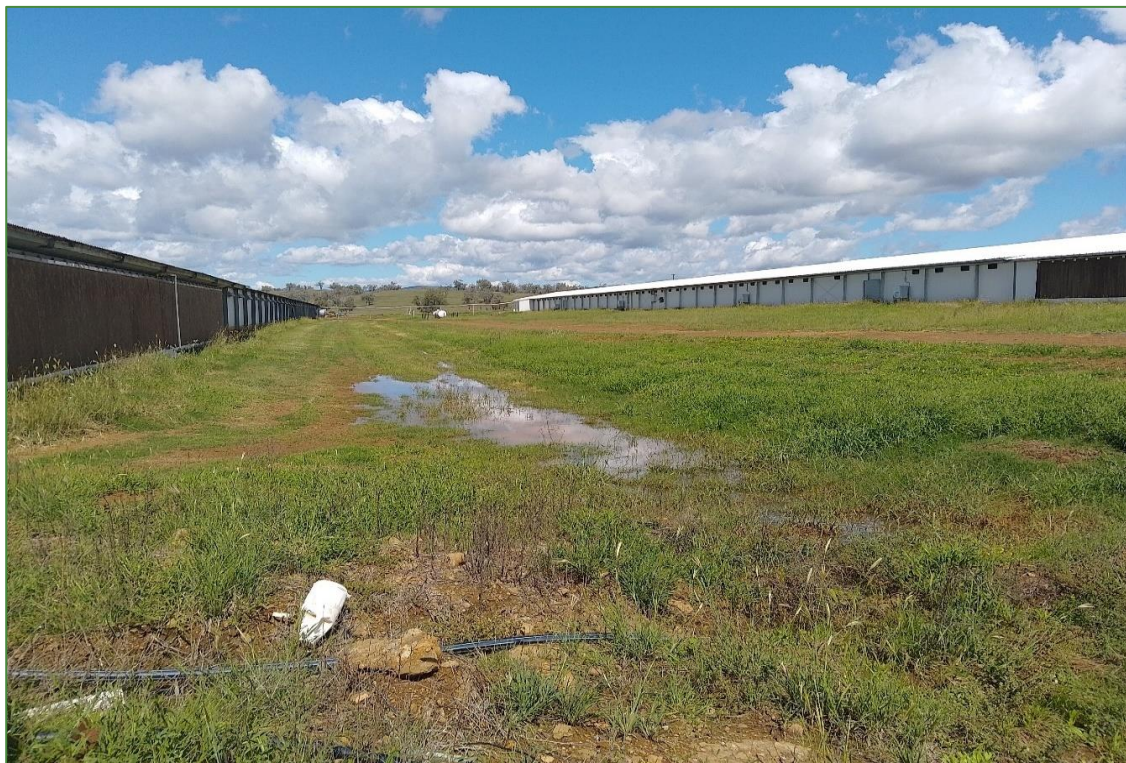
Photograph 4: Between sheds (viewer is facing S)
