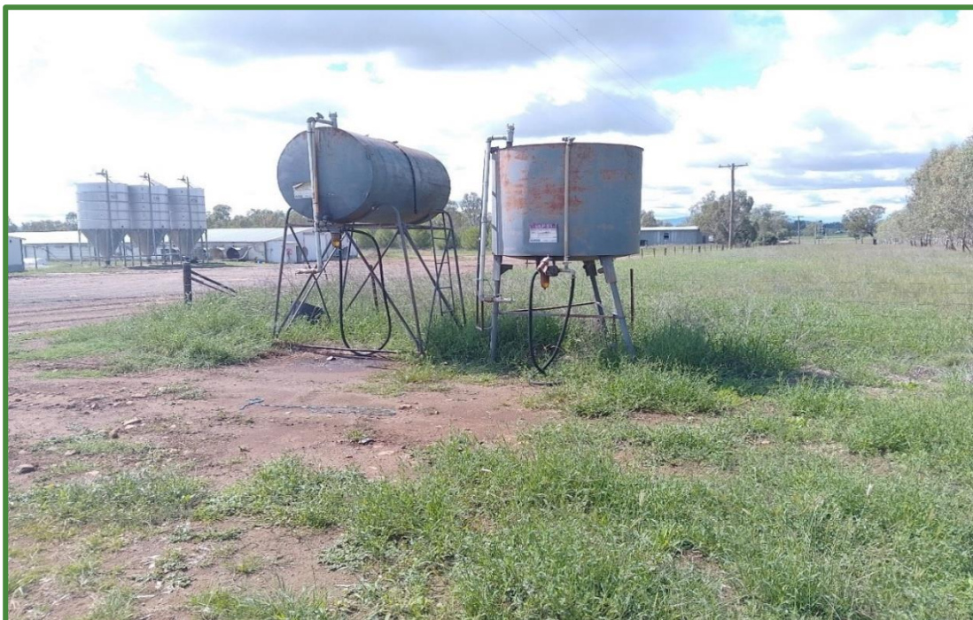
Photograph 8: Diesel/Petrol Tanks (superficial surface contamination beneath bowser)
