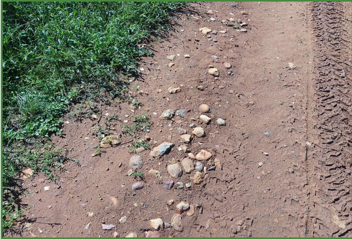
Photograph 15: Close up of typical side of driveway
